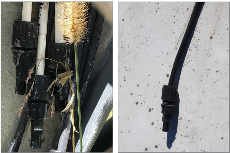
The connectors above are examples of potential time bombs: they were left unplugged without end caps at a utility-scale plant (left) and a commercial rooftop system (right).
