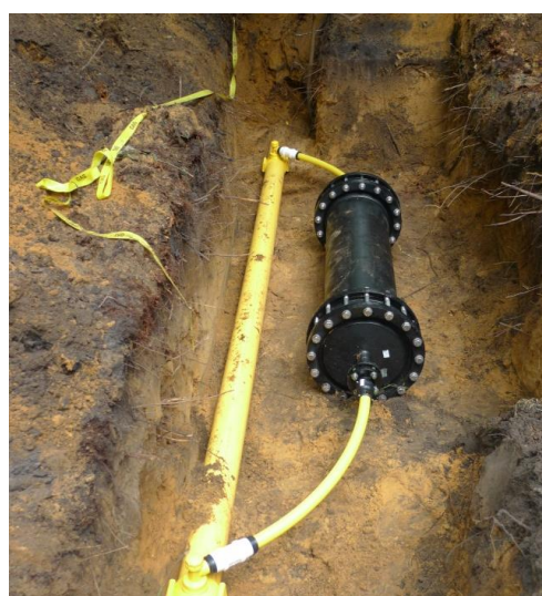
Figure 16. Test rig under G-gas conditions.
